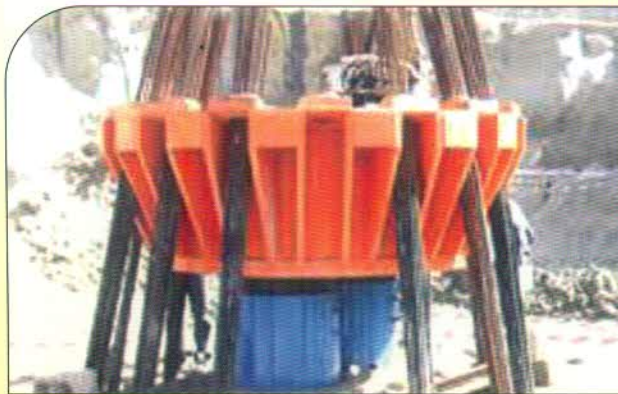
Pile Load Testing By Rock Anchor Method
