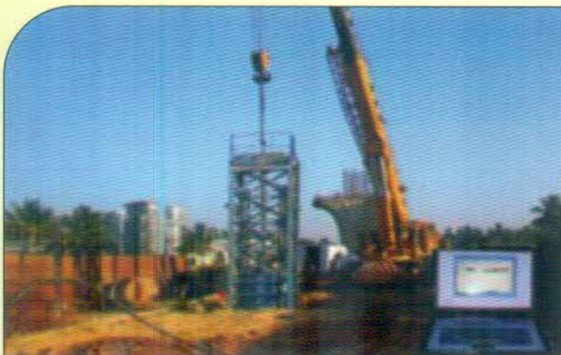
High Strain Dynamic Pile Load Testing
