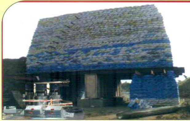
Pile load Test By Kentledge Method
