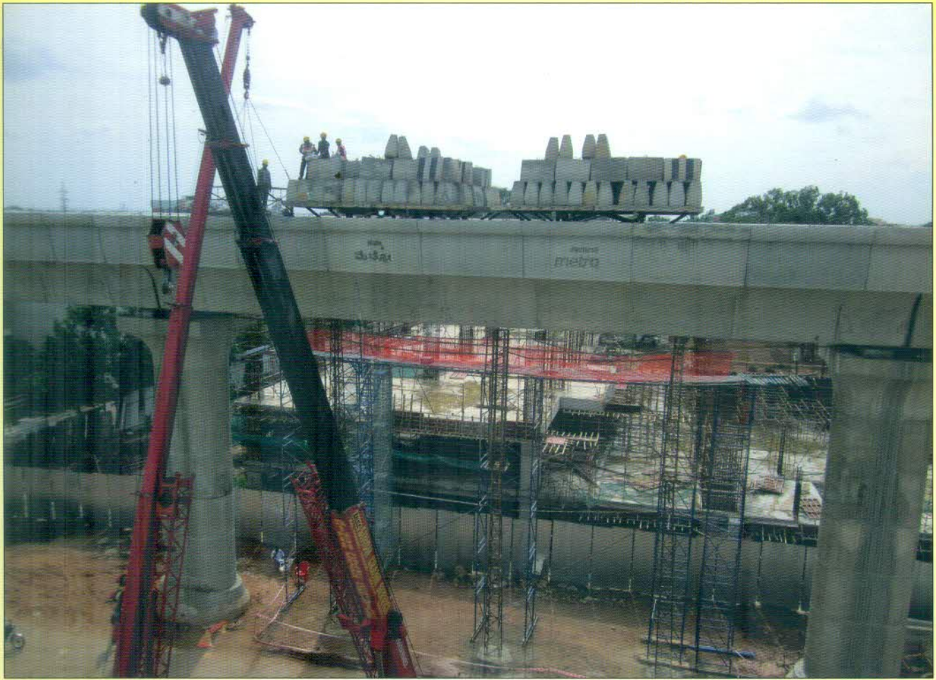
Span Load Testing of Metro Rail - Viaduct
