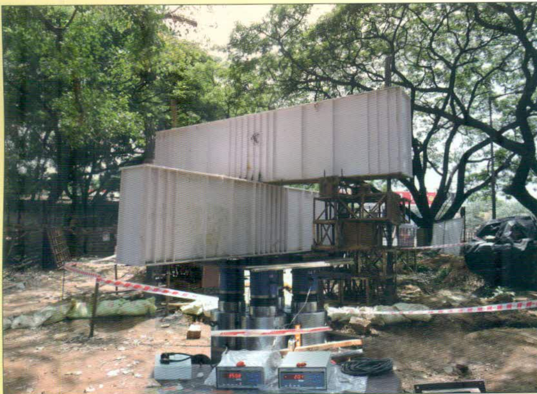
Pile Load Testing
